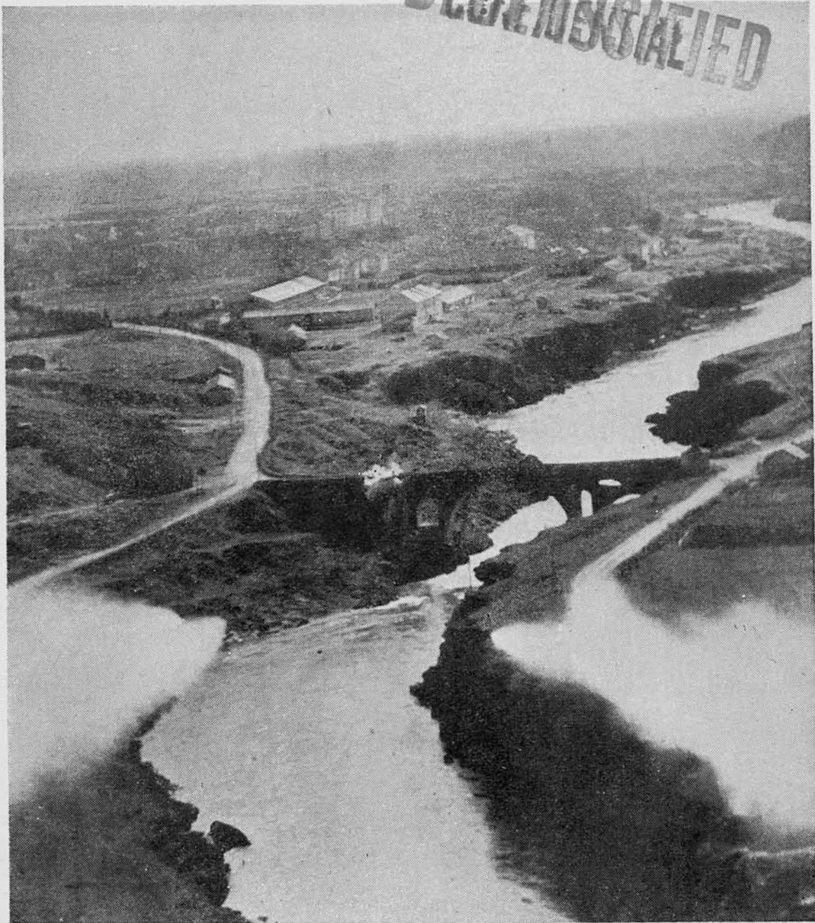
A bridge near Gorica under attack by S.A.A.F. Beaufighters. Note damage from preceding aircraft.
